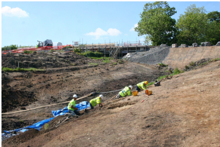
Excavation of a prehistoric burnt mound on the course of the A40 Penblewin to Slebech road scheme
